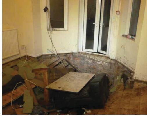
(ABOVE) THE DAMAGE DONE BY STUDENT REVELLERS DANCING ON ROTTEN TIMBERS
